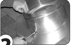
Align roof pitch number on elbow on peak of roof as shown. Position straight with the indicator line on the base flashing. and mark hole to be cut. Locate rafters by Place 3 screws through holes that line up tapping roof. with predrilled holes in base.
